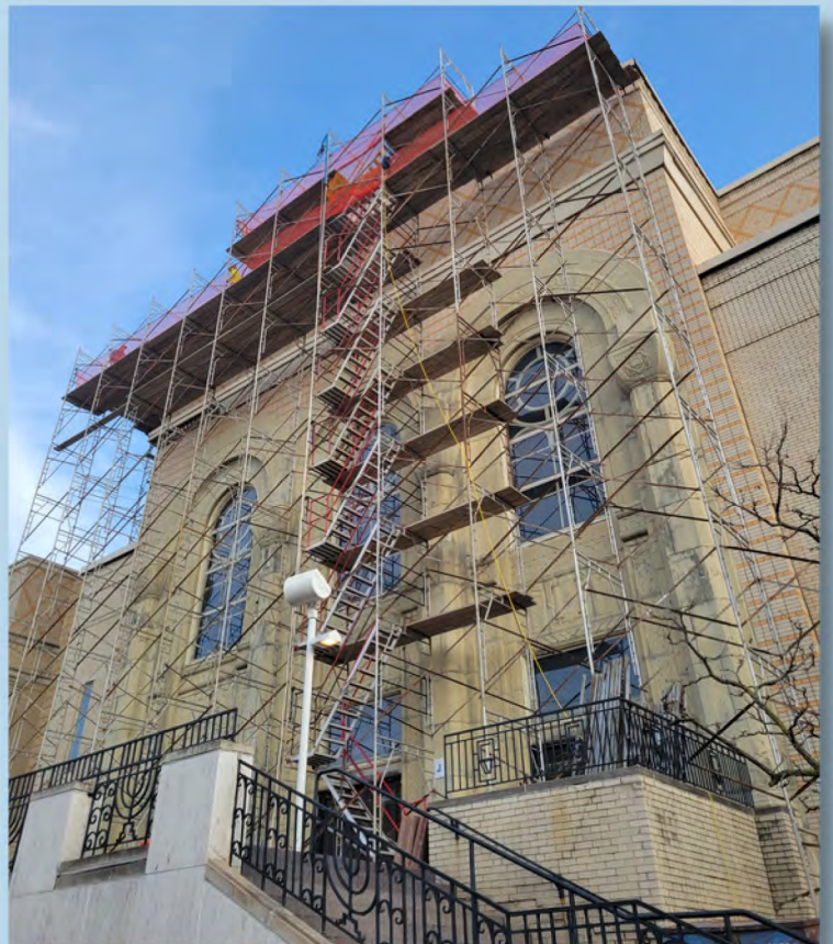
Cornices being replaced around the entire sanctuary building
