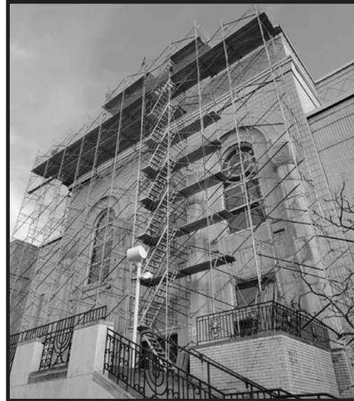
Cornices being replaced on side of building on Beacon Street
